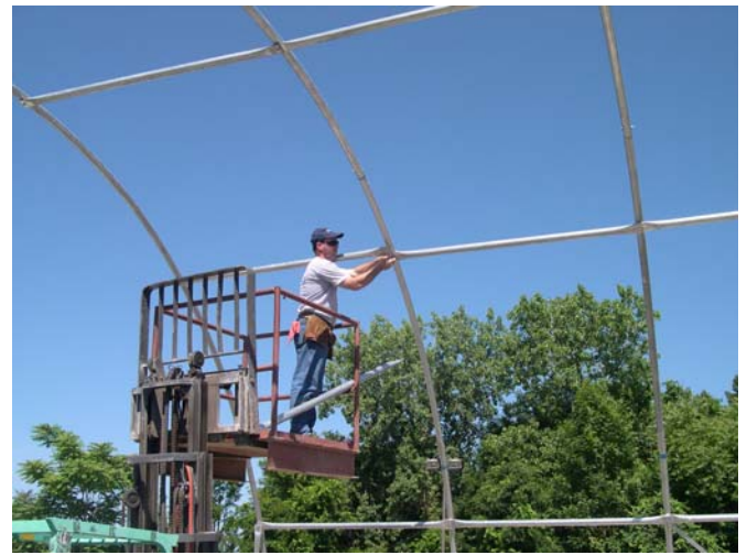
Cross Rails Inside Connect Arch Assemblies
