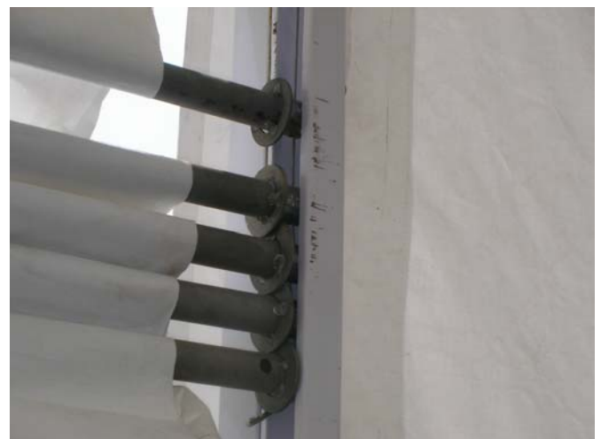
Door Tubes Inserted Into Door Track
