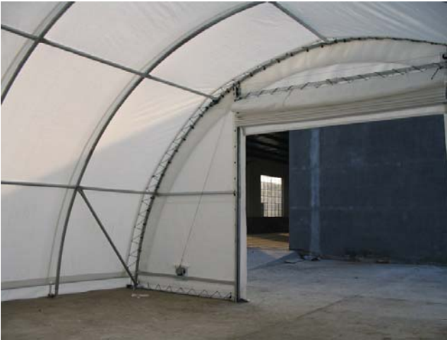
Main Roll Up Door in fully Open Position
